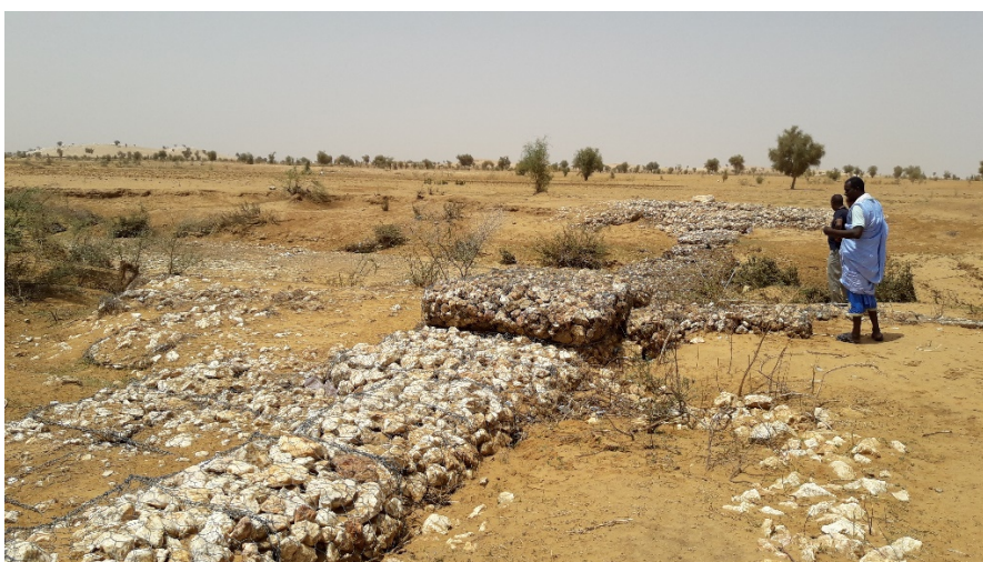
Figure 7: Beilougue Litama Block dam, installed 2014, still functioning, cropping area with shrubs in background (time 11.38.05)
