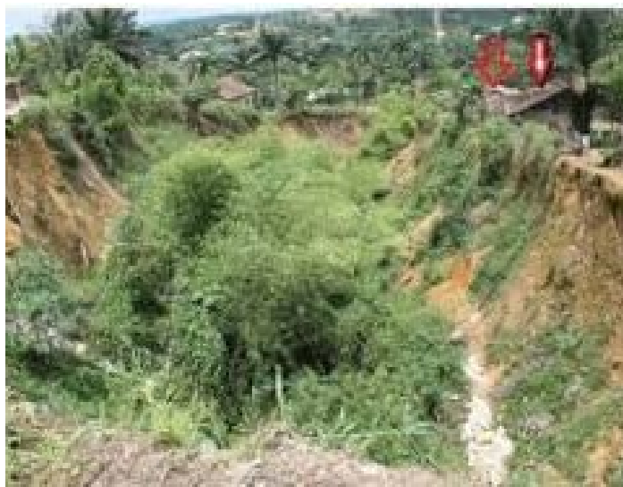
Ikot Ekpo site in Cross River (Before)
