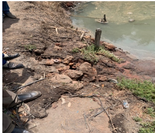
Dyke repair by local communities
