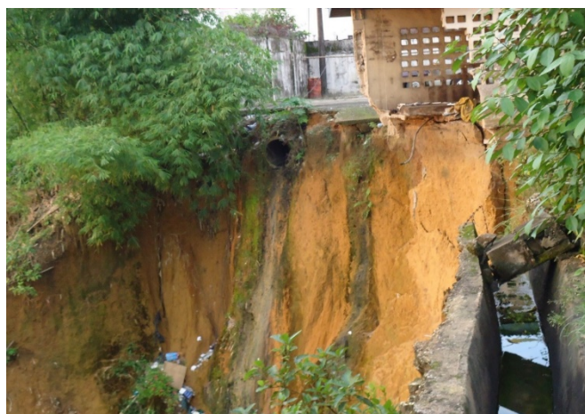
Atakpa site in Cross River State (Before)
