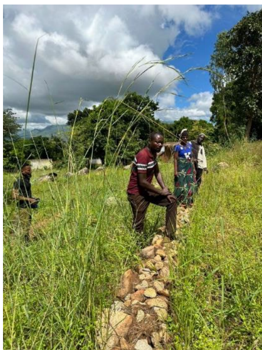
Catchment area management through stone bunds, vertiva grass and swales trapping water
