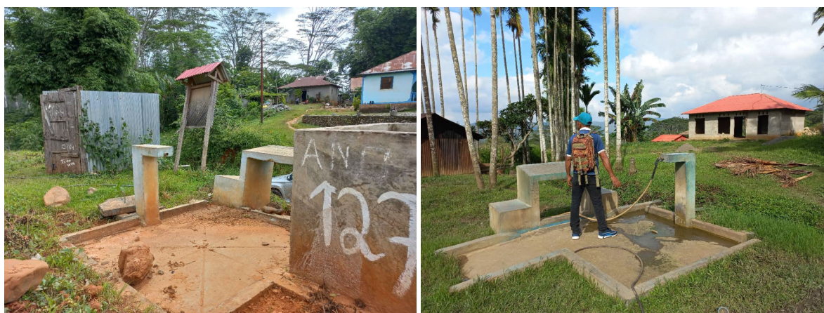
Photo 7: One water collection point that has stopped working (left) and another one that is fully operating near the water source (right) in Talimoro (Ermera)
