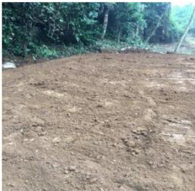
Contaminated soil was compacted with vibrating tamper
