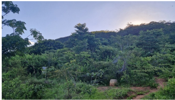
Gully control through gabions and plants in water run-off area
