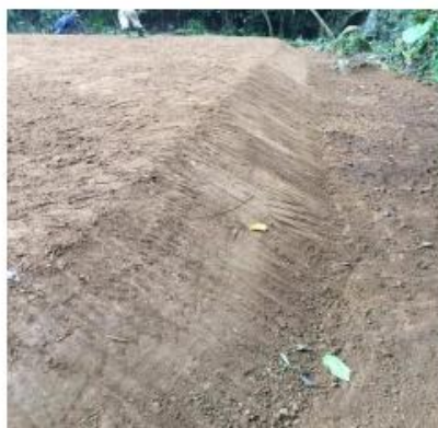
Surface was covered with clean soil and compacted
