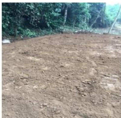
Contaminated soil was compacted with vibrating tamper
