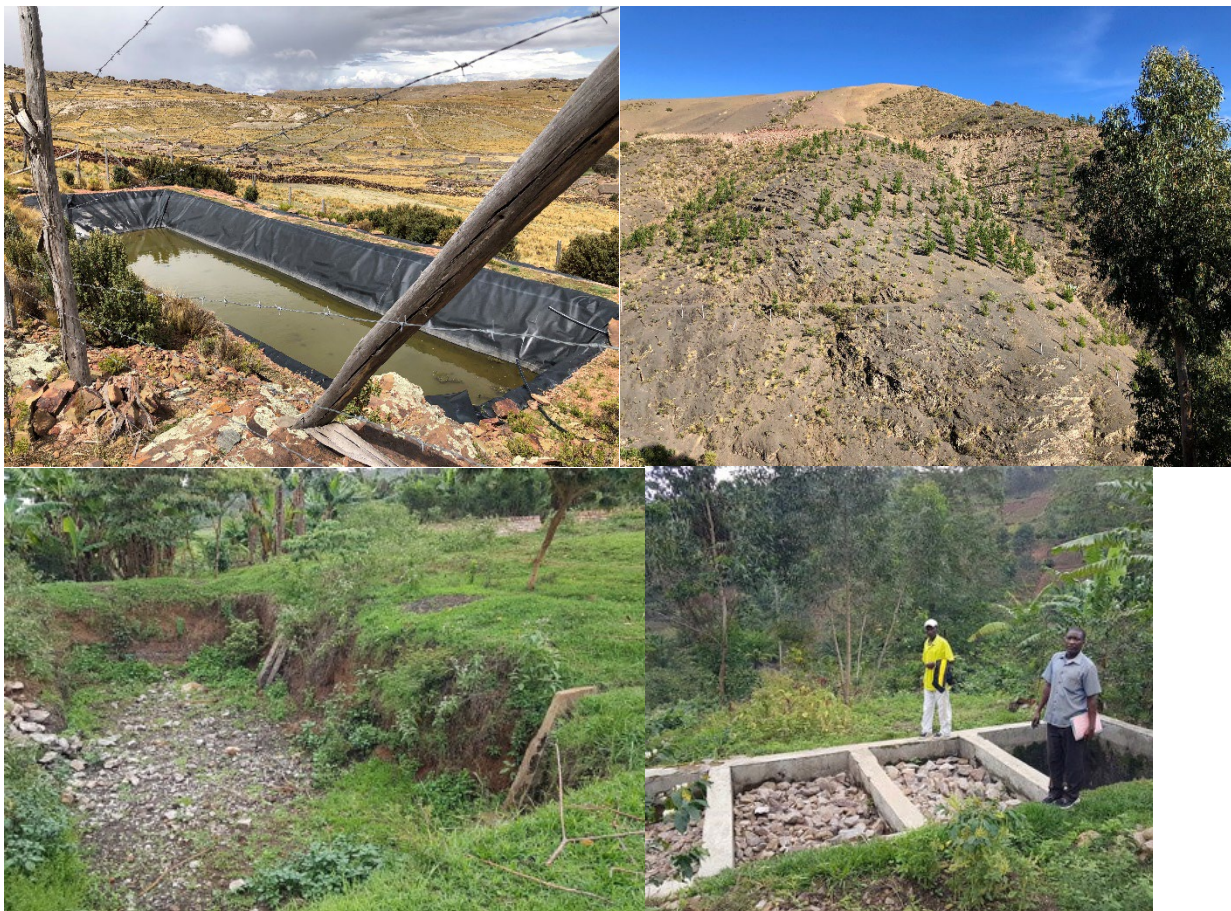
Figure 10. Photos showing sustainability of GEF project activities relating to water security. Top photos show an intact geomembrane and tree plantation installed by the Bolivia EVAs project in Walkeri and Chekene communities in 2016-17. Lower photos show coffee washing infiltration ditch and treatment tanks installed by the Burundi PROZOC project in Mwiro and Burunga communities in 2015-17.
