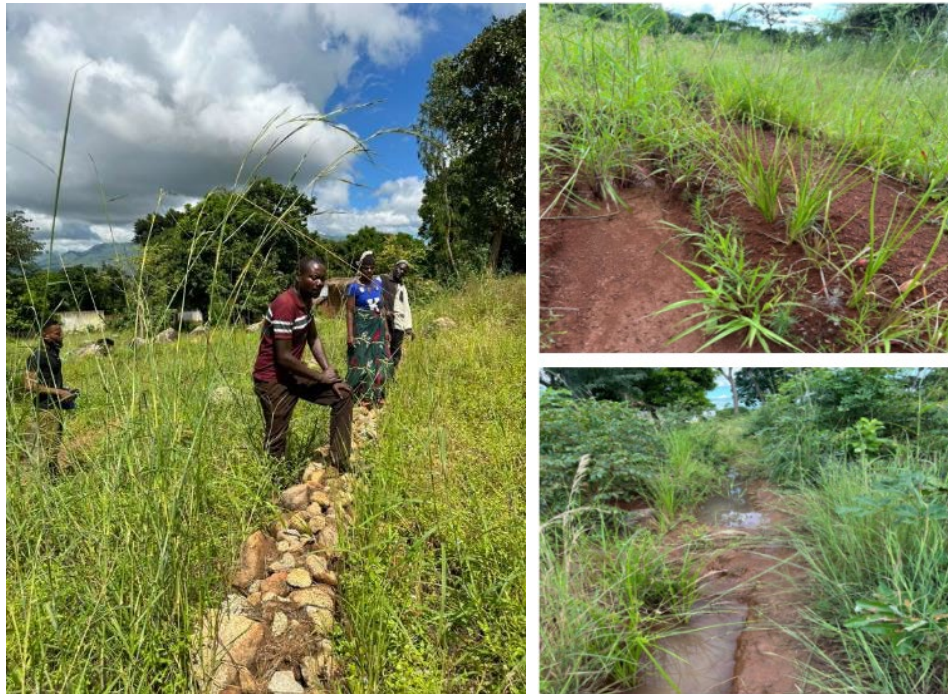
Catchment area management through stone bunds, vertiva grass and swales trapping water
