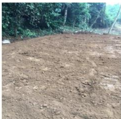
Contaminated soil was compacted with vibrating tamper
