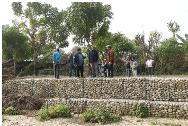
Nepal: Check dam with vegetation reinforcement for flood protection
