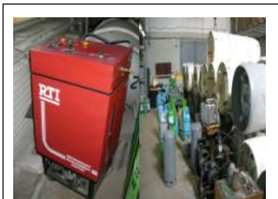
Figure 31: RTI recovery and recycle equipment (left) and stored ODS (right). Revers Refrigeration, Latvia.
