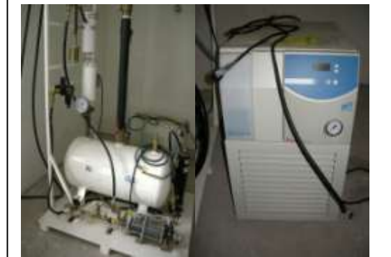
Figure 25: Little-used halon recovery and reclamation equipment. Polygon Research Centre, Kazakhstan.
