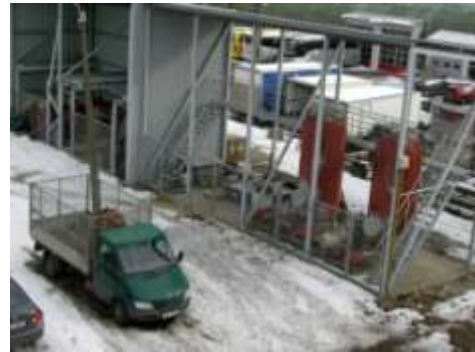
Figure 11: Halon decommissioned from ships using truck and small crane, with storage tanks in background. Halon Bank, Estonia.
