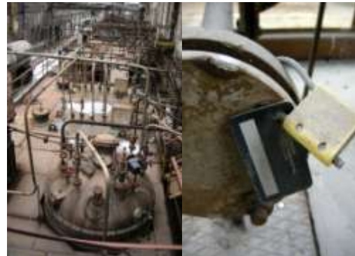
Figure 52: Disused CFC production plant (left) and sealed CFC production pipe (right).
