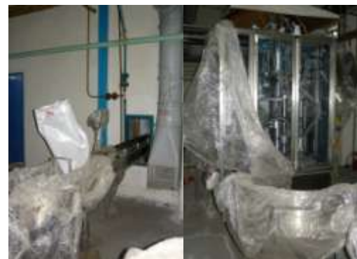
Figure 51: Connection to exterior for hydrocarbons (left) and valve filling equipment (right), both in storage under plastic. Chimprom Aerosols, Volgograd.
