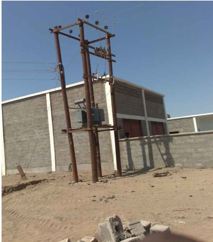
Photo: Completed powerhouse and grid reticulation at the project site
