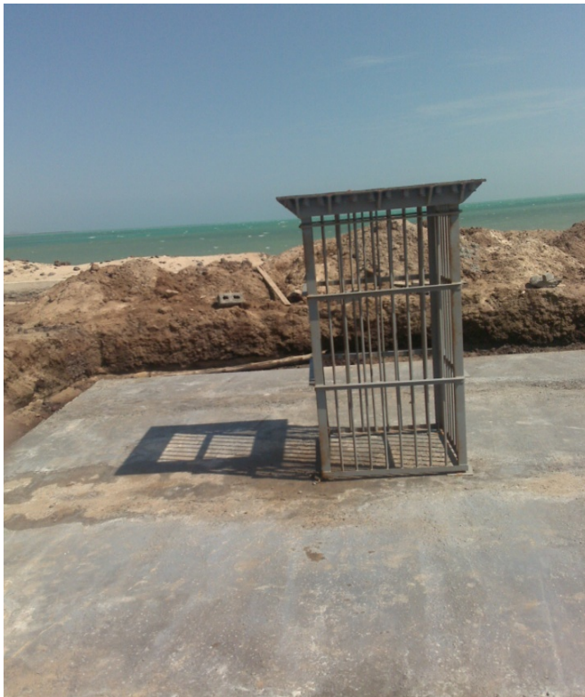
Photo: DoE modified platform design for the distributed wind system showing removal of redundant bars and the design of an elevated platform and widened foundation (to accommodate high water levels due to the proximity to the sea) accepted by contractor
