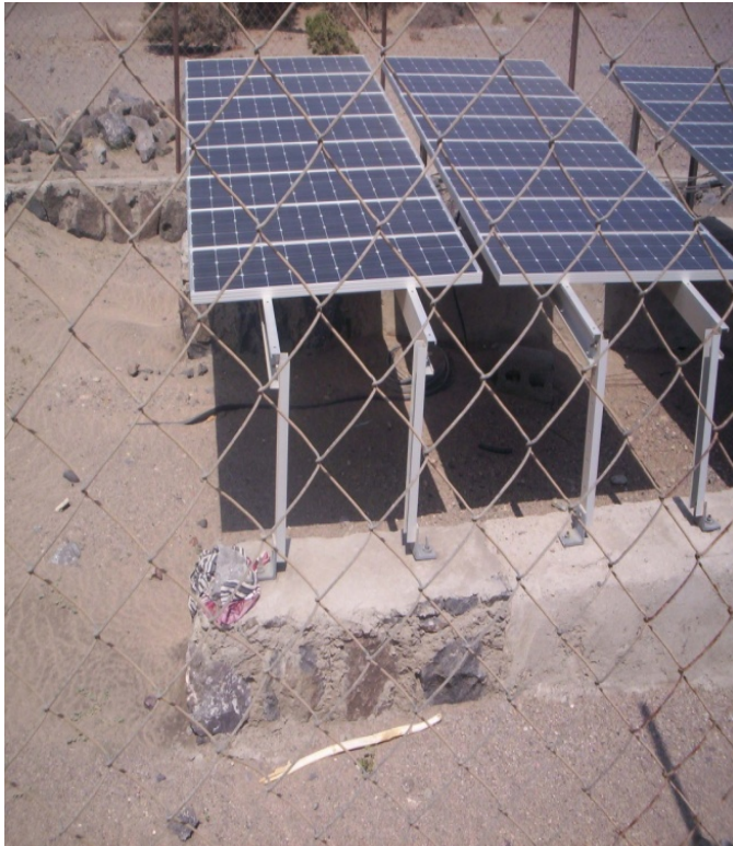
Photo: Solar System for Water Pumping – ERTC data has been instrumental in installation of solar for water pumping
