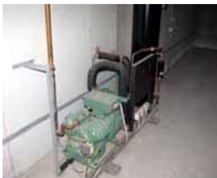
Figure 9: New Danfoss R-404 compressor at Linda Ltd.
