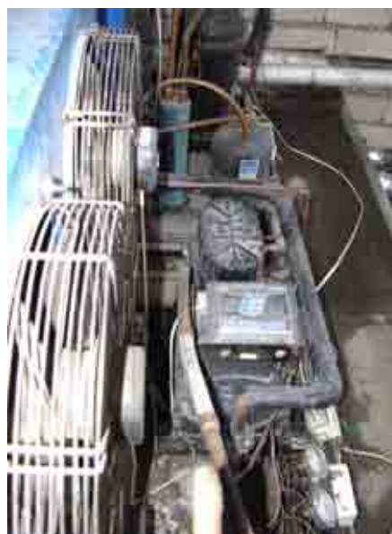
Figure 8: New Copeland R-22 condensing unit at Daroink
