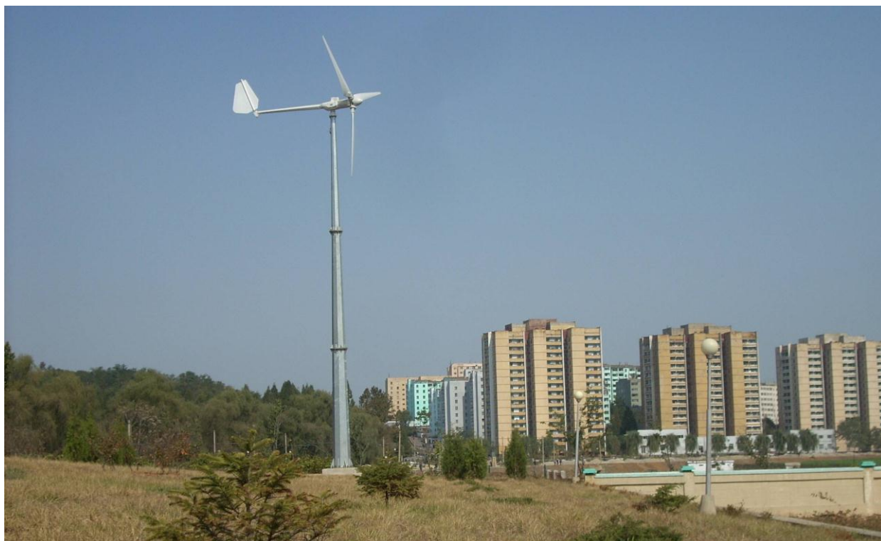
Commercial 5-kW wind turbine as part of a hybrid (wind-PV) electricity backup system for the hospital at Unjong County.
