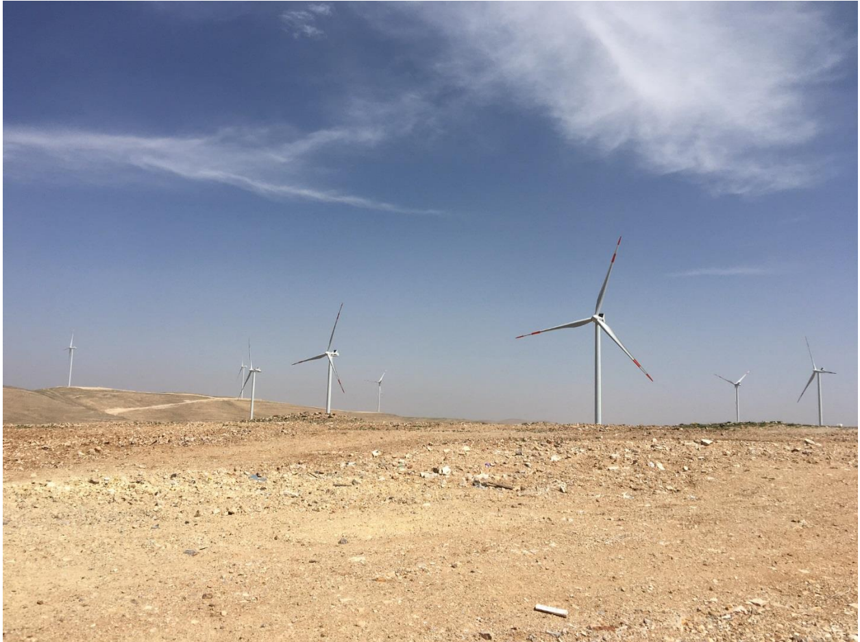
Figure 12.1. Northwestern part of the Tafila Wind Farm (Source: World Bank staff; Site Visit 03/08/2016).
