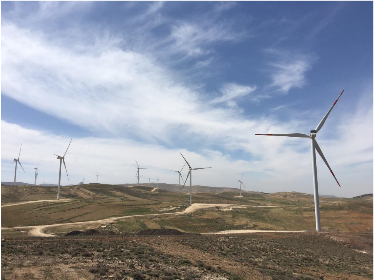
Figure 12.2. Southern part of the Tafila Wind Farm (Source: World Bank staff; Site Visit 03/08/2016)
