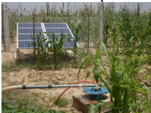
Solar-powered irrigation of a corn and millet field
