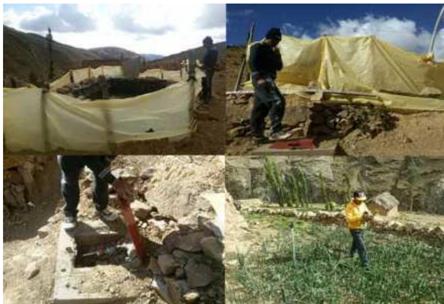
Figure 27. Micro irrigation system built with the support of the EVA project. A) water reservoir B) Chamber C) Water valve and D) Sprinkler delivered by the project.
