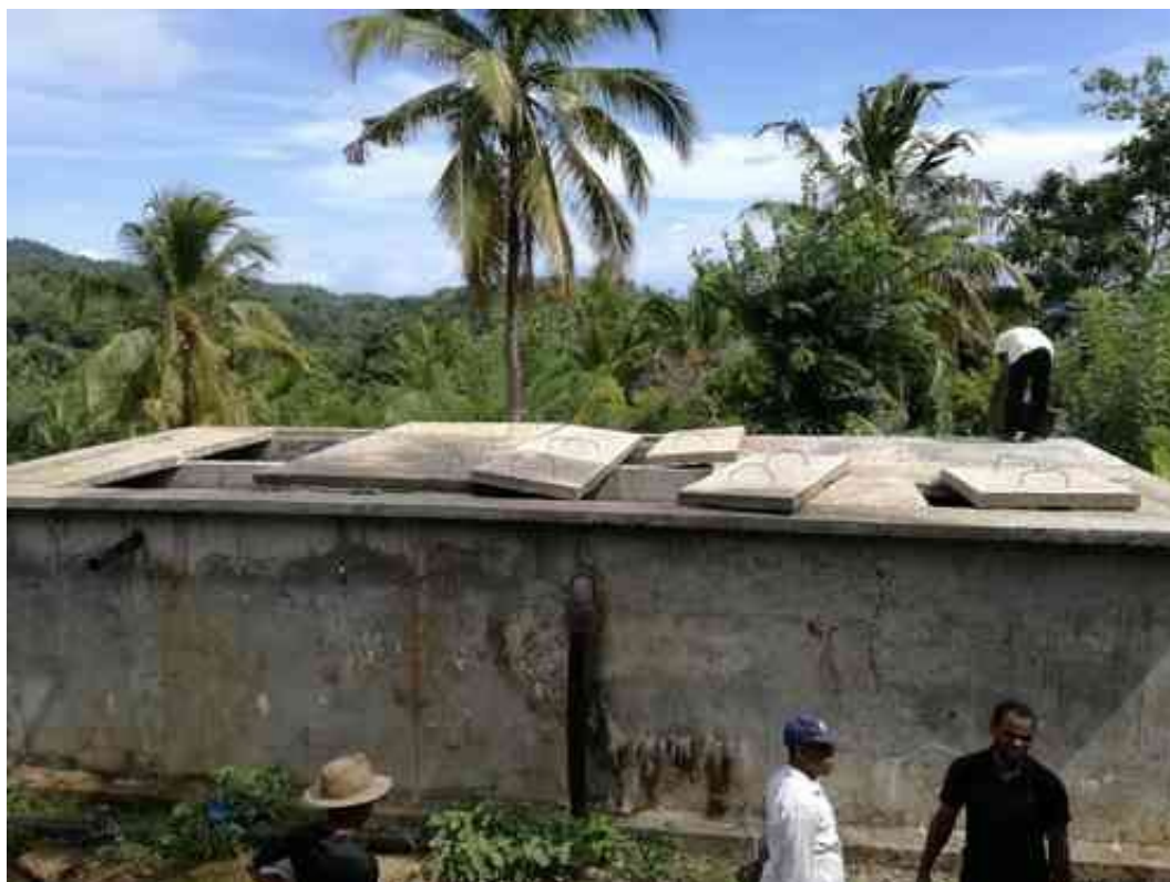
Slow Filter, Lingoni-Hoani water supply scheme. The covers turned out to be too heavy to manage. The plan is to substitute them with lighter covers.
