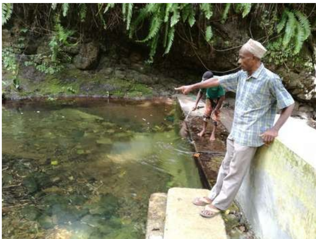
Rehabilitated intake, Lingoni-Hoani water supply scheme
