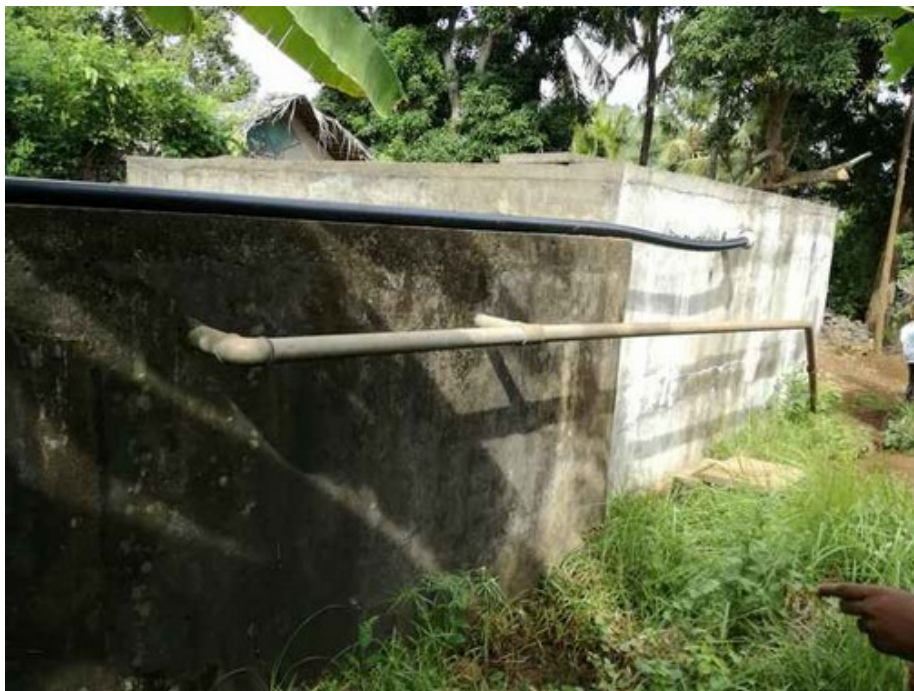
Lingoni-Mbatsé water supply scheme. New (right) and old (left) water reservoir. As the new reservoir has few connections, it overflows into the old reservoir (black, upper pipeline) making more water available for the existing distribution system.
