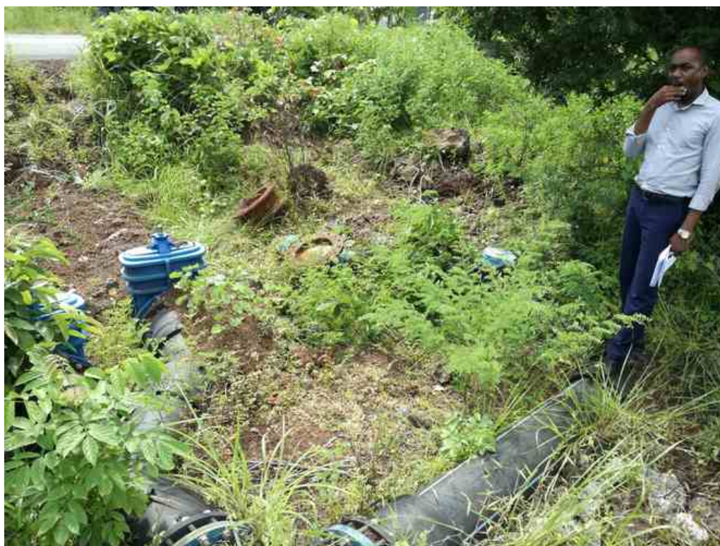
Airing valve, Moroni water supply project.
