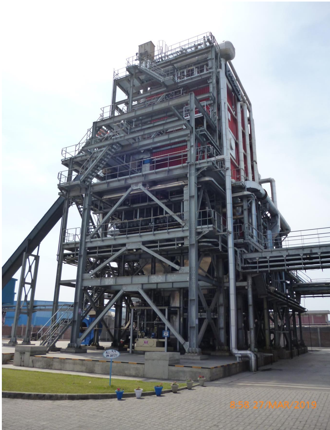
Figure 2: Sapphire Finishing Mills' Boiler for 5.5 MWe Biomass Plant Showing Boiler Scale
