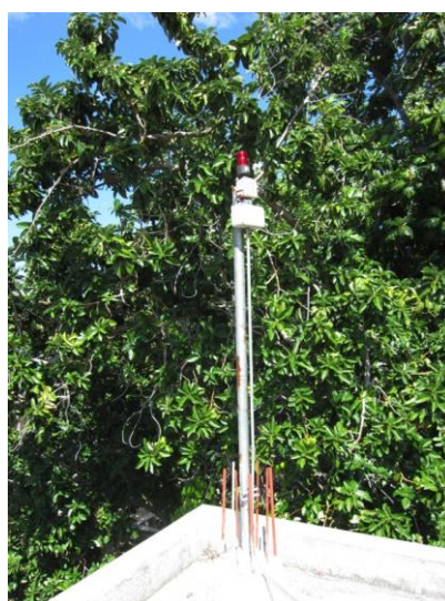
Image 18: Burglar alarm to protect solar panels. Port-à-Piment.
