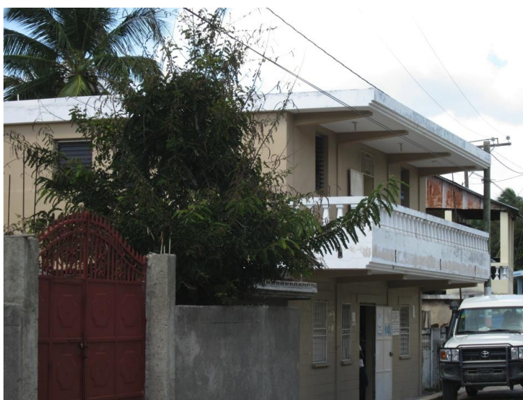
Image 24: Dispensary. Solar panels on top of flat concrete roof. Roche-à-Bateau
