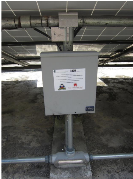
Image 20: Twin inverters providing 6KW. Port-à-Piment.
