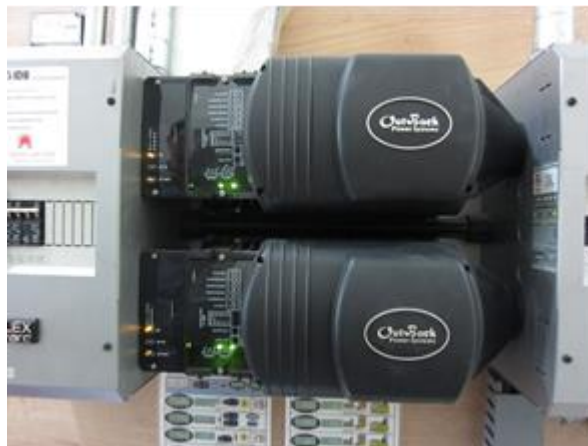
Image 20: Twin inverters providing 6KW. Port-à-Piment.
