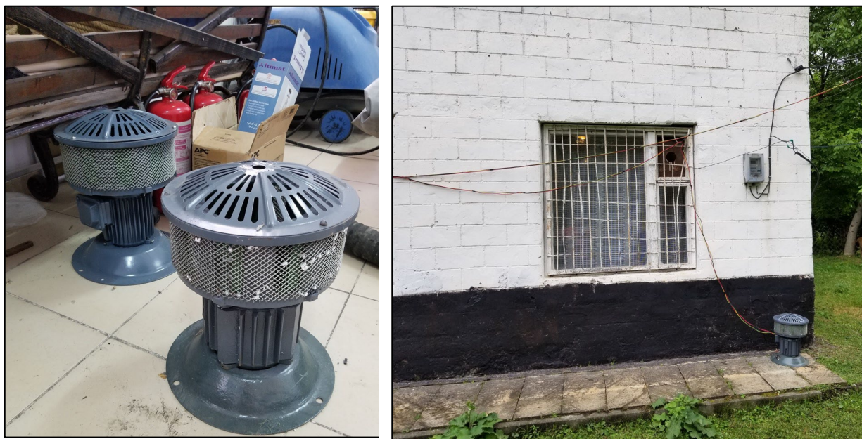
Figure 12 Emergency Sirens for Flood and Landslide Disasters and Early Warning System
