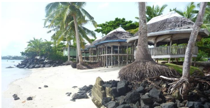
Figure 2.1 Beach erosion, failed attempts to stop it with rocks and a retaining wall, and the vulnerable beach fale on the north coast of Savaii
