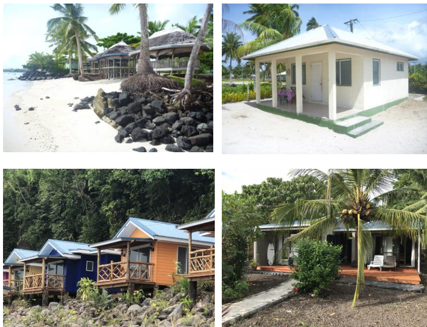
Figure 3.6 The progression of fale improvement delivered by the Project's Small Grants Program: Top Left – at risk light build beach front fales, Top Right – Phase One response that delivered resilient but less authentic buildings, Bottom right – the introduction of design and larger fales containing ensuites, Bottom Left – large scale relocation and replacement of fales with inbuilt design
