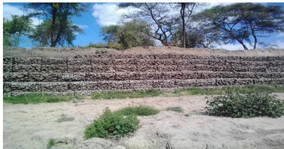
Figure 1: Ume River Gabion constructed: Protecting riverbank undercutting to save school from destruction.
