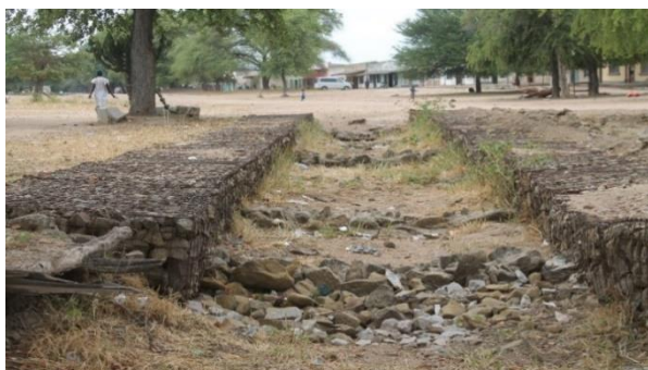
Figure 2: Gabions and silt traps protect waterway below Business Centre. Silt trap controls velocity and erosive power in the hospital gully downslope.
