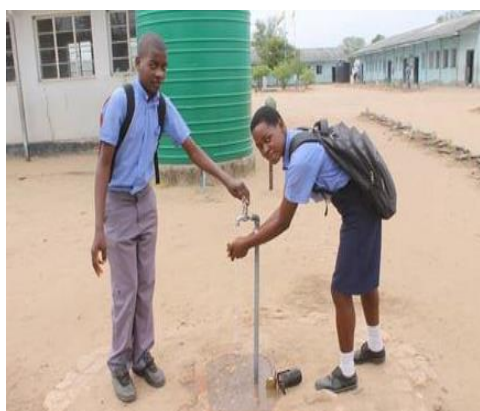
Figure 7: Roof rainwater harvesting in the middle catchment through a network of 64 tanks at two Schools and the Hospital to control gully erosion downslope. Tanks also serve as a garden water source. Taps are locked to avoid water wasting by pupils.
