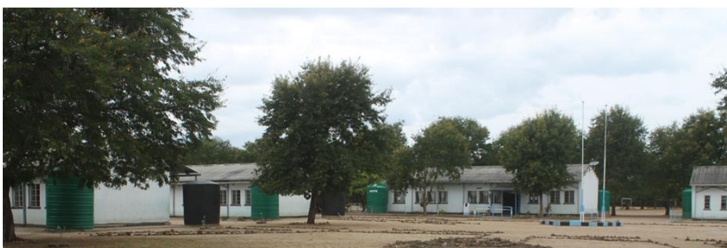
Figure 6: Roof water harvesting tank network at Chireya Secondary school for reducing and retaining runoff to control gullies downslope.
