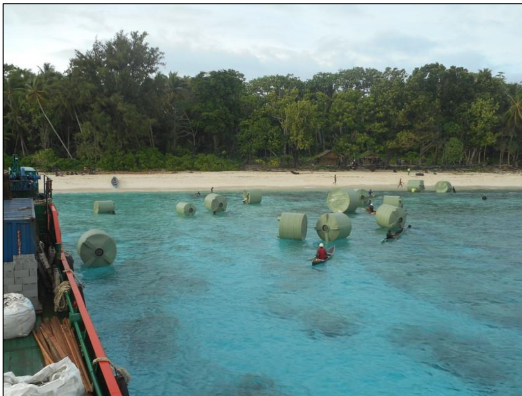
FIGURE 5: Rainwater tanks being floated ashore and guided by canoes after delivery by cargo ship to Aurigi (Santa Catalina) Island. The extremely remote nature of many of the project sites presented significant logistical challenges to timely delivery of project outputs, and the original budget did not account for the high cost of sea-freight in the Solomon Islands. This is a lesson for project budget planning in future project designs (image: SIWSAP)
