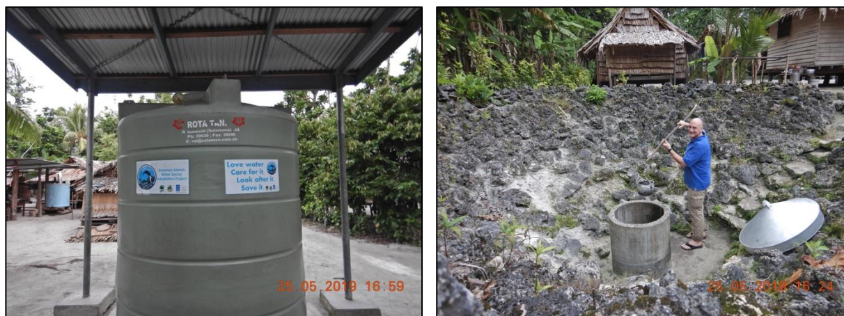
FIGURE 8: The main boost to water security and resilience from SIWSAP has been from the installation of rainwater tanks (left) and the rehabilitation of groundwater wells (right) (source: Raaymakers)
