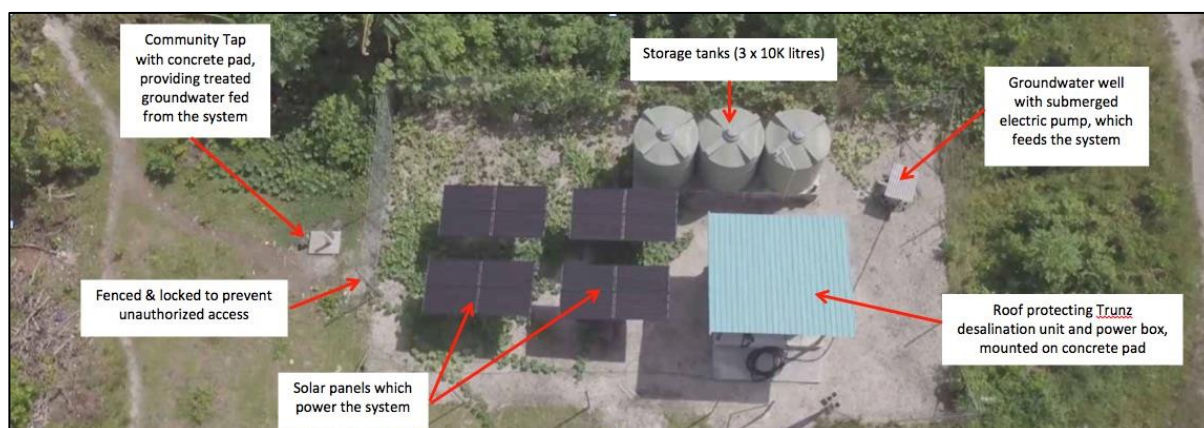
FIGURE 7: An example of one of the Trunz solar-powered groundwater desalination system and associated storage tanks, reticulation pipes, community taps and associated infrastructure (this one at Taro) (source: SIWSAP)
