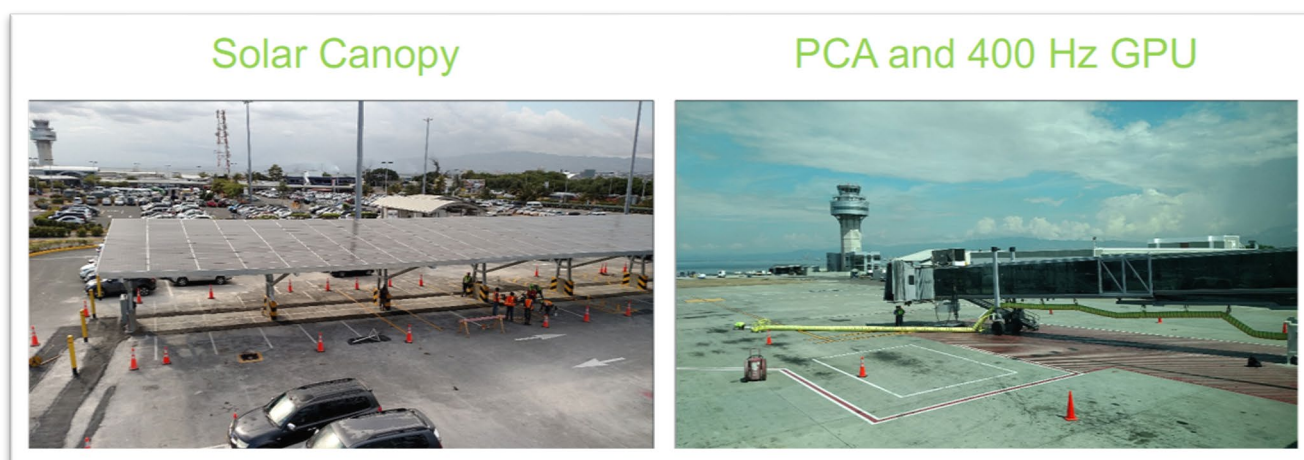
Figure 13: Photos of the 100KW Solar PV array under construction and Gate 1 with the PCA and GPU. Note the air traffic control tower behind the solar array in the upper left of the photo. Source: ICAO
