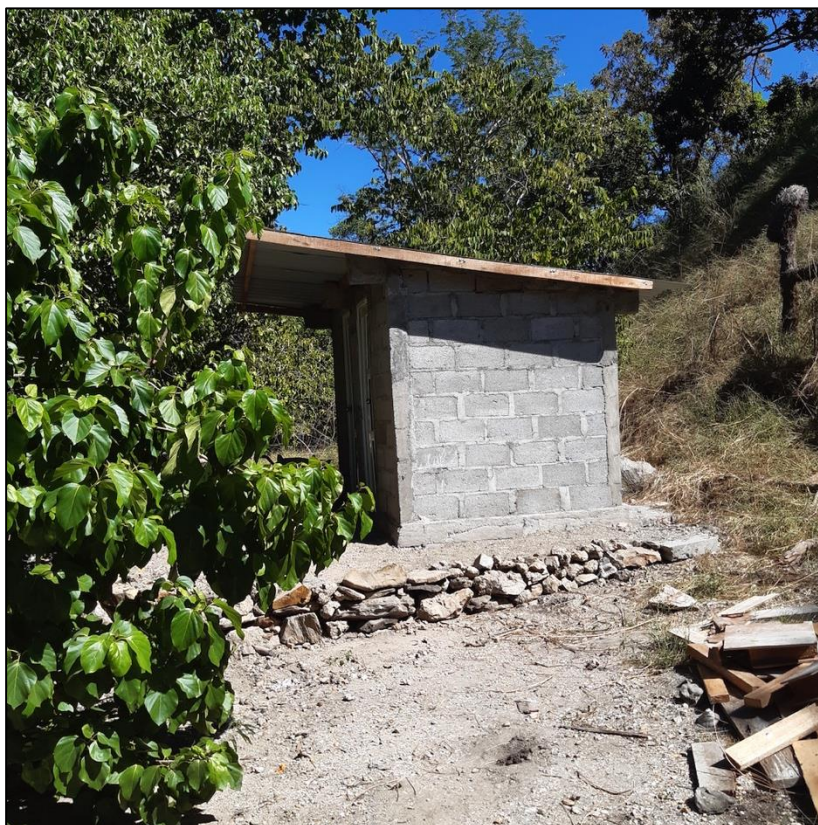
FIGURE 11: The toilet block installed by the CRB project at the eco-tourism site in Hera. Reportedly this is completely non-functional due to lack of water supply from the tank shown in Figure 12. Note also the poor construction standards and building debris left lying around the site (bottom right) – which is not acceptable for an ‘environmental’ project. This is an example of poor design, planning and construction oversight by the project (image: da Costa)
