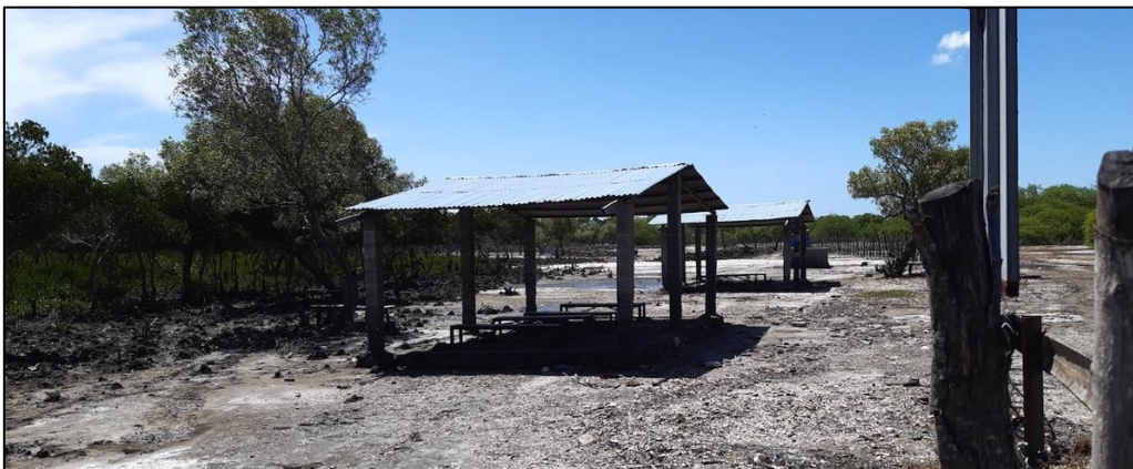
FIGURES 7A & B: The failed BBQ fish stalls built by the project in Metinaro without proper market analysis and business planning. The top image clearly shows the very poor design standards and low quality, non-durable building materials used. These do not represent ‘resilient infrastructure’ – which is supposed to be a key focus on the CRB project. They are also located right on the mangrove fringe, in an area that could be better suited to re-afforestation (NOTE: during the same time period other community-developed BBQ kiosks along the roads both east and west of Dili were conducting brisk business – NC Pers. Obs.) (images: da Costa)
