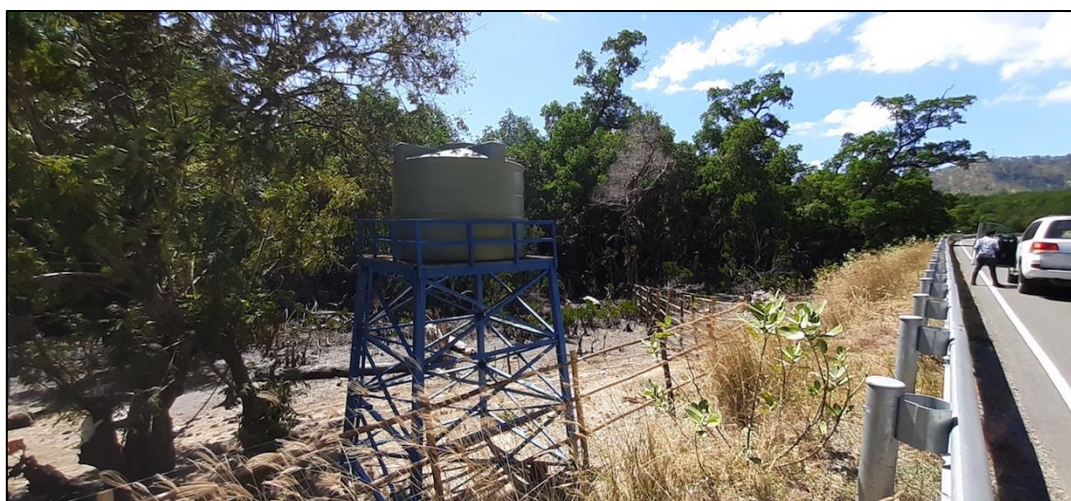
FIGURE 12: The water tank installed by the CRB project at the eco-tourism site in Hera to supply the toilet block shown in Figure 11. Reportedly this is completely non-functional because is not sited correctly to allow gravity-fed water supply. This is another example of poor design, planning and construction oversight by the project (image: da Costa)
