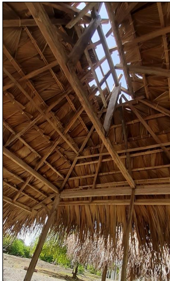
FIGURES 10A & B: The uncompleted and now abandoned eco-tourism facilities built by the project at Wenunuk in Metinaro. Apart from illustrating the waste of GEF funds by not being completed and utilized, the bottom image shows the non-durable materials and low standard of construction methods (images: da Costa)
