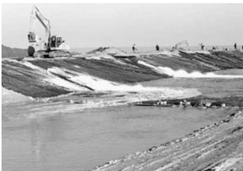
A canal, 12 kilometres long, 40 metres wide at the top and 20 metres wide at the bottom, has recently been dug (People.net, 18 February 2002)
