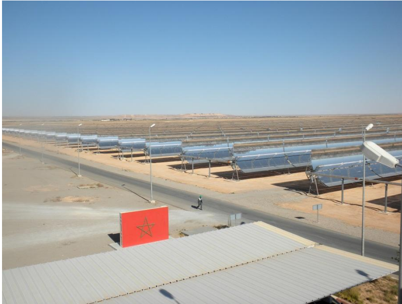
The Ain Beni Mathar ISCC solar field – June 2012
