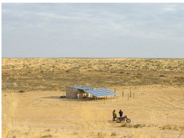
Figure 10: Solar Panel Installation
