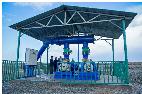
Figure 8: Installation of Water Intake Pumps
