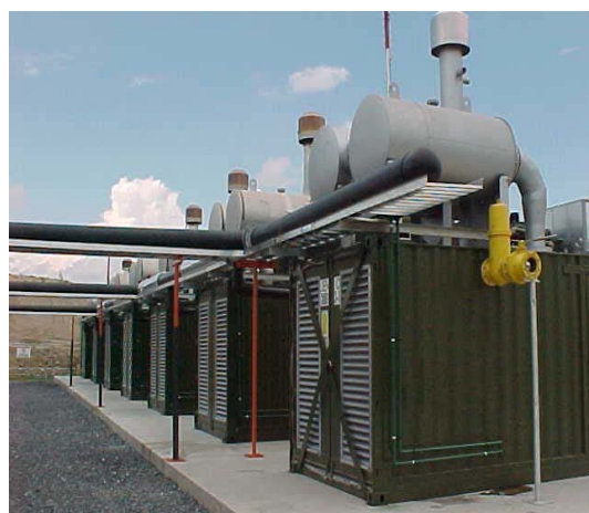
Figure 11: Motor-Generators
