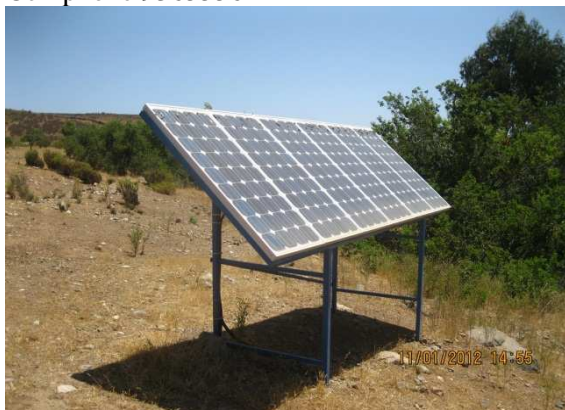
Generator which consists of 6x75 Wp (= 450 Wp) ISOFOTON modules IS-15S/12
