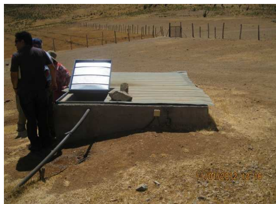
Storage tank of 7 m³
