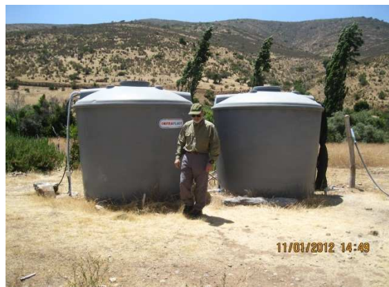
Storage tanks of 10 m 3 (m 3 2x5)
