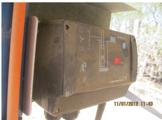
GRUNDFOS pump system regulator
