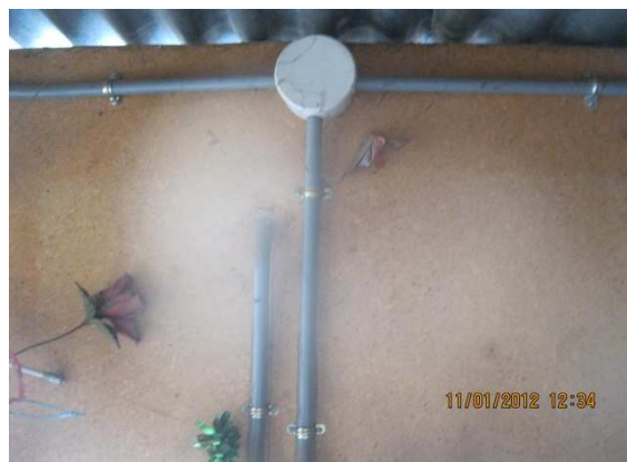
Detail installation with wiring in electrical PVC pipe
