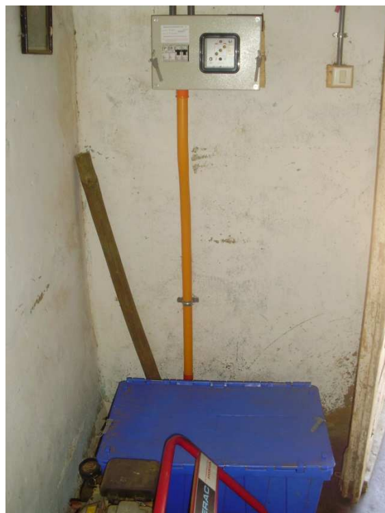
Battery box. Keep watch to prevent user access to the battery
