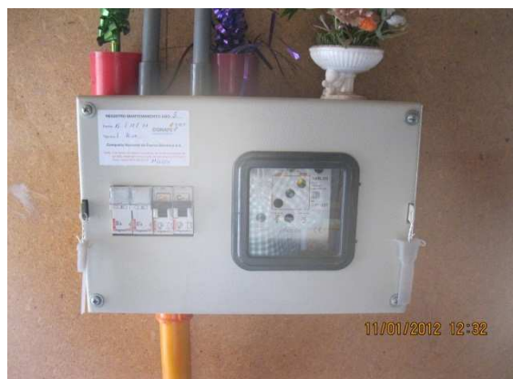
Box with charge regulator (Phocus) (right center) and breaker (left center). Sticker of system review by CONAFE. 150 Ah wet-cell deep-cycle batteries, base-mounted metal.
