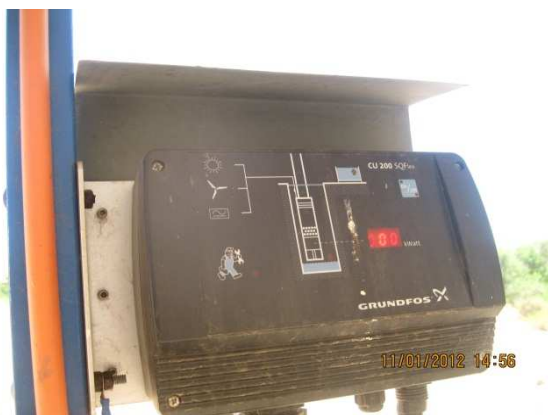
GRUNDFOS pump system regulator
