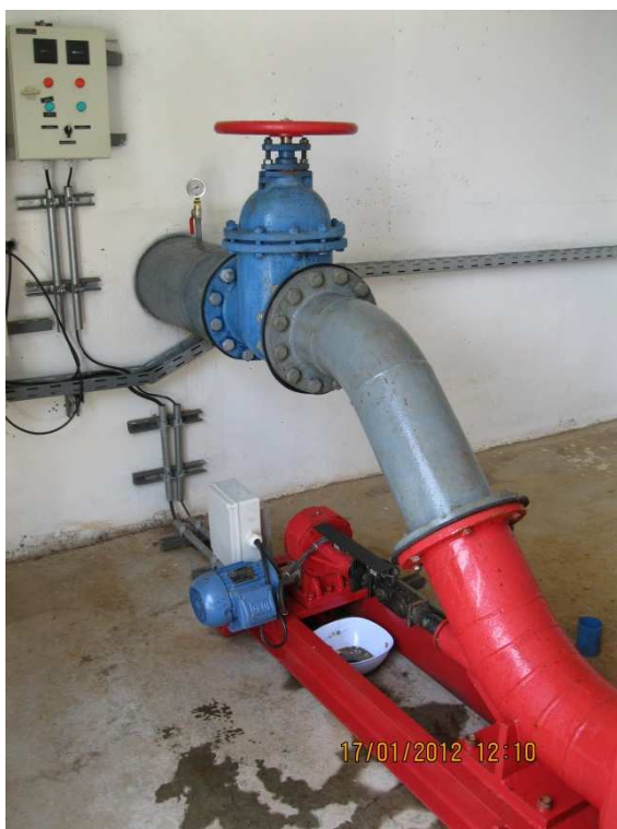
Penstock, valve and regulator
