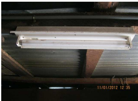
Luminaire installed at 12 VDC
